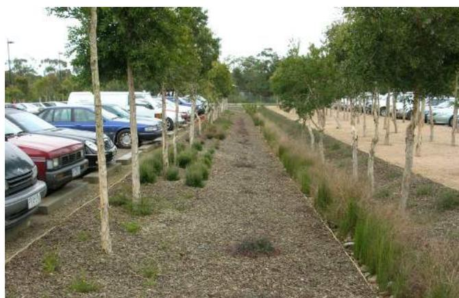
Locating a naturally vegetated swale within a car park increases visual amenity whilst providing passive infiltration.
