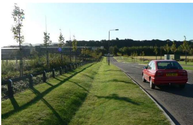
A grass channel incorporated into the road verge will passively treat stormwater run-off.
